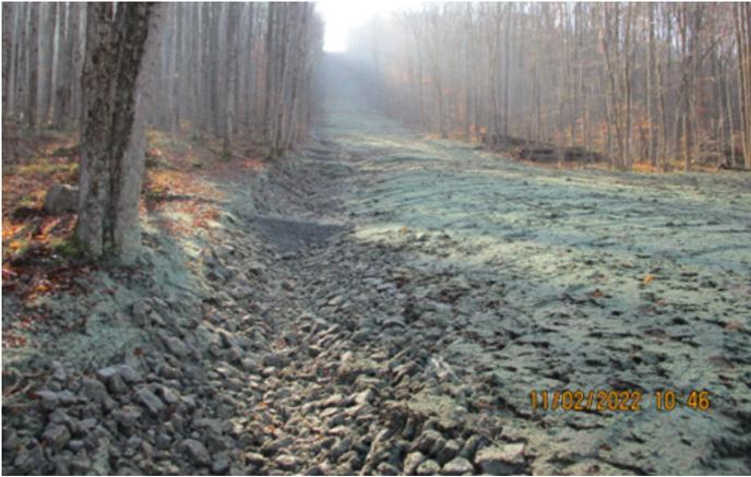
*Stormwater channel installation and ROW stabilized with hydromulch application*
