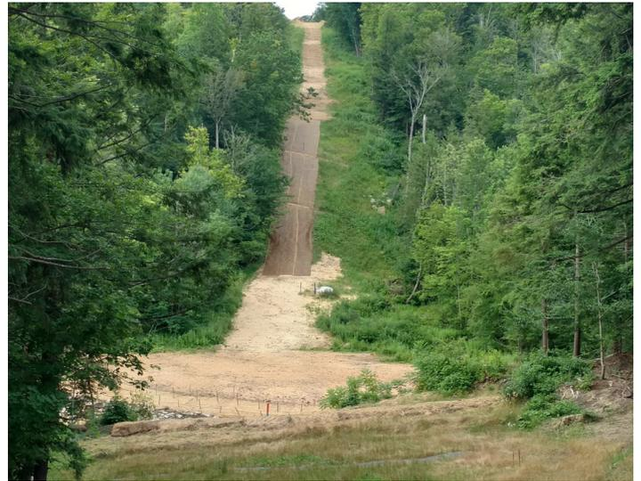
*Water bar installation to minimize erosion on a steep slope*
