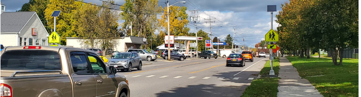
The Washington St. Road Diet project in Watertown, NY, reduced pedestrian accidents 90% in a busy corridor housing three schools.
